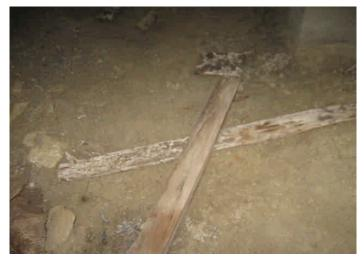
Some of the pier posts did not have damage to the concrete base pads due to the high moisture content in the soil, due to the compartmental design of the areas under the home and the hillside moisture condition, there is inadequate ventilation in the crawlspace under the home, recommend further evaluation by a qualified foundation specialist for corrections and upgrades.
