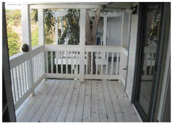
Deck and stair railings current construction requirements are for 42 inches in height which is a recommended upgrade in structures built before 2008, however, a requirement in structures 2008 and after. *Components and Conditions Needing Service*
