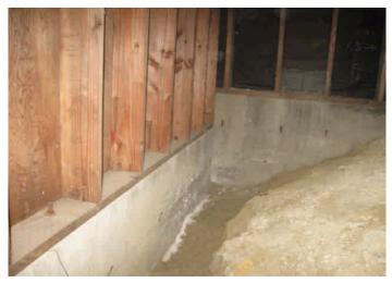
The pier posts under the structure were not strap anchored to the beams which was acceptable at the time the building was built and are recommended to be upgraded to have metal t-straps screw anchored across floor stringer beams to the vertical pier posts.
