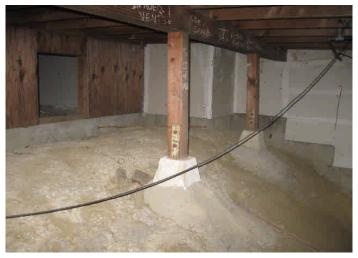
Wood or cellulose debris has been left under the structure and is recommended to be removed. Refer to the termite inspector for further evaluation and corrections.
