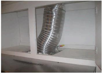
The range hood has been improperly wired with exposed connects not properly installed in a junction box, recommend corrections by an electrical specialist.
