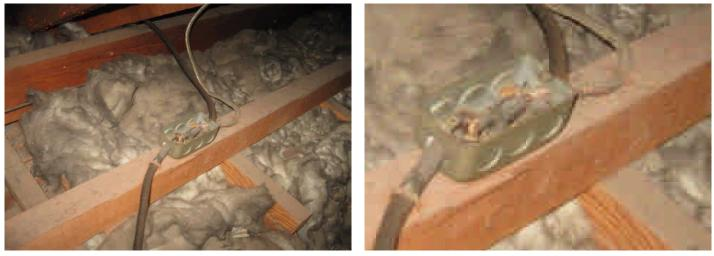
Obsolete and suspect knob and tube wiring is present within the attic, which should be inspected and certified as safe, or replaced by a licensed electrician.
