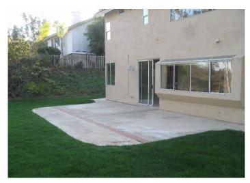
The patio concrete has been improperly installed close or over the stucco weep screed flashing, it does appear to have slope directing water away from the walls and no evidence of moisture intrusion was found at the time of the inspection, however, moisture intrusion will remain a possibility, monitoring for moisture intrusion is recommended and particularly during rainy weather to verify no moisture intrusion is occurring.
