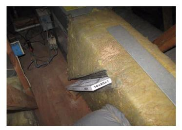
Filters for the forced air system were dirty and are recommended to be replaced.
