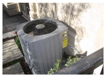
Recommend strapping the AC condenser to the base pad to prevent accidental movement that might damage the refrigerant or electrical power lines.
