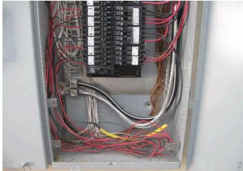
AFCI bedroom breakers to prevent arcing are in place in the main panel. These are to prevent arcing at electric outlets and plug in items in the bedrooms that might cause arcing\spark fires. If no power in the bedroom electric outlets, it is recommended that you check for any sources of electric sparks in the bedroom and reset the AFCI breaker in the electric panel.
